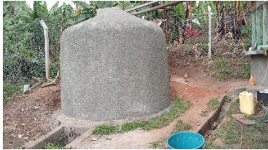
Figure 5; Complete renovated water tank
